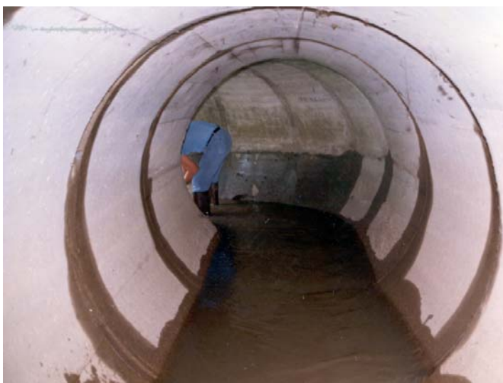
FIGURE 2: Typical Joint Infiltration in Non-Gasketed Storm Sewer
